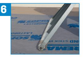
Use a membrane roller to apply pressure over the entire membrane surface to ensure full adhesion.
