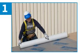
Unroll the membrane horizontally, making sure it is properly aligned.
