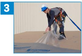
Remove the film at a 45° angle so as to avoid wrinkling.
