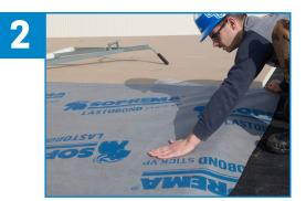
Remove a portion of the silicone release film and adhere the end of the membrane.
